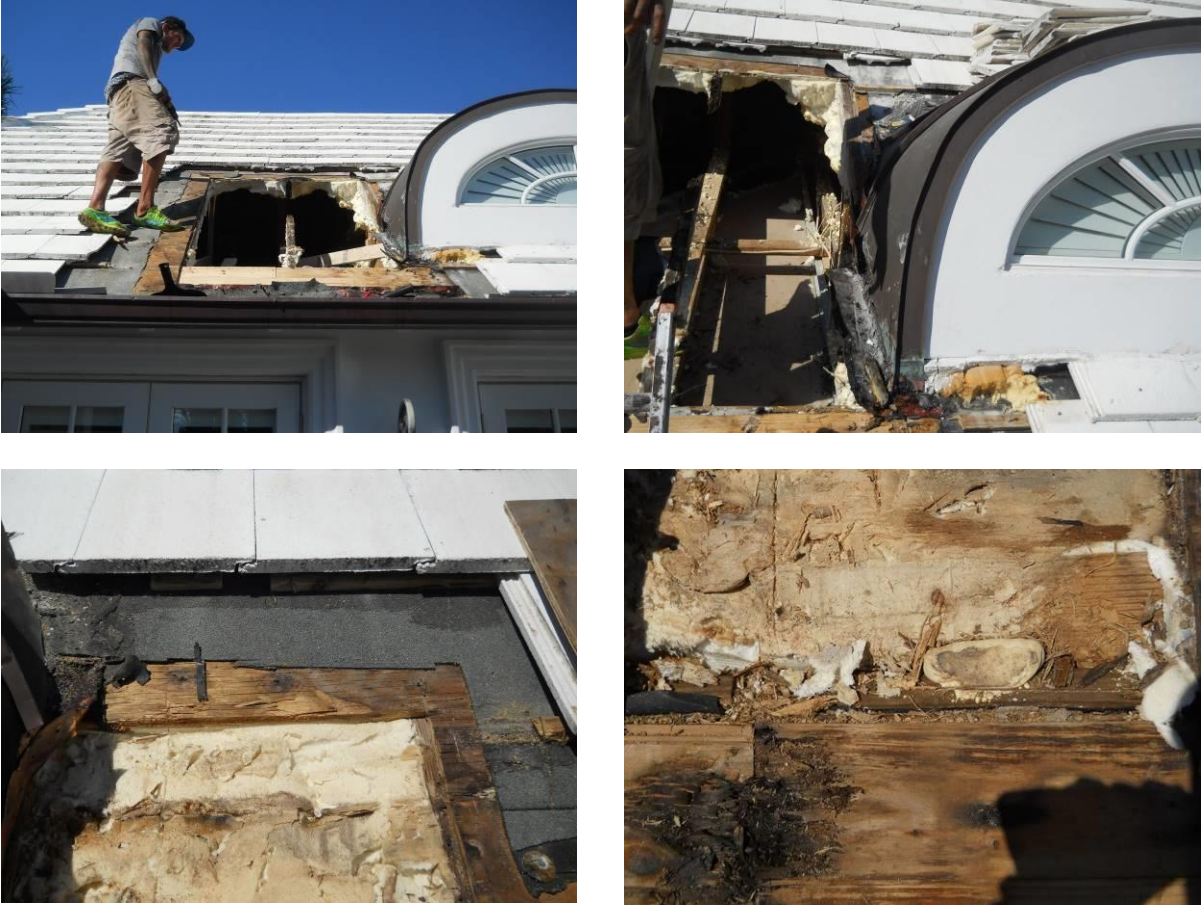
Figure 8: Moisture damage in an unvented attic with ccSPF. Moisture was particularly event around the visible dormer (Courtesy of Mark Zehnal).
