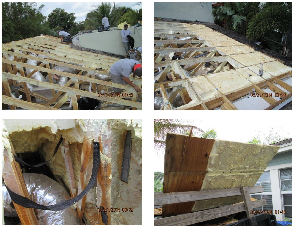
Figure 10: Evidence of moisture buildup in home installed with ccSPF. Note the moisture on both the sheathing and wood framing
