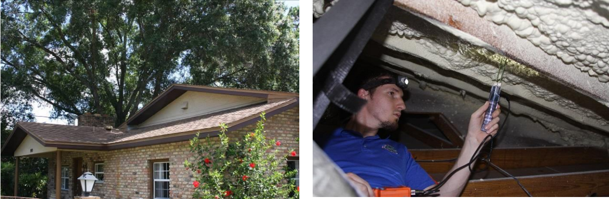
Figure 12: (Left) View of the front of the house from ground. (Right) View from inside the attic showing the ccSPF and a moisture content measurement being taken.
