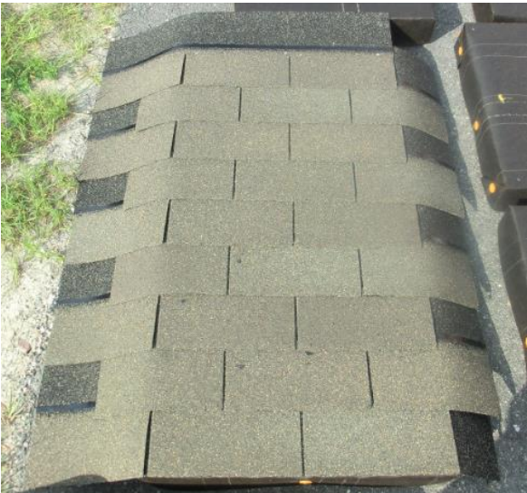
Figure 32: Membrane installed on all edges to prevent uncontrolled moisture travel
