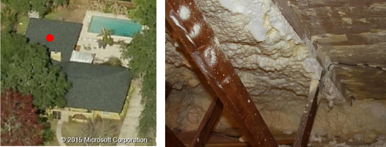
Figure 13: (Left) Aerial view of Home 2. The red dot indicates the approximate location of the photo to the right. (Right) ocSPF installed in the attic space. The truss shown is directly over the garage wall. SPF to the right of the truss, over the garage, has been removed by the homeowner.
