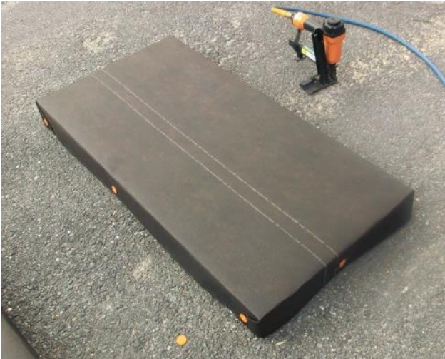
Figure 32: Membrane installed on all edges to prevent uncontrolled moisture travel
