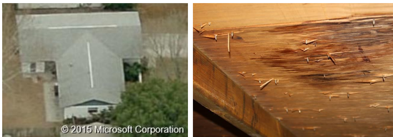
Figure 14: (Left) Aerial view of Home 3; (Right) Apparent water damage in the plywood sheathing. No moisture was present at the time of inspection, and no evidence of past moisture was evident in the insulation below.
