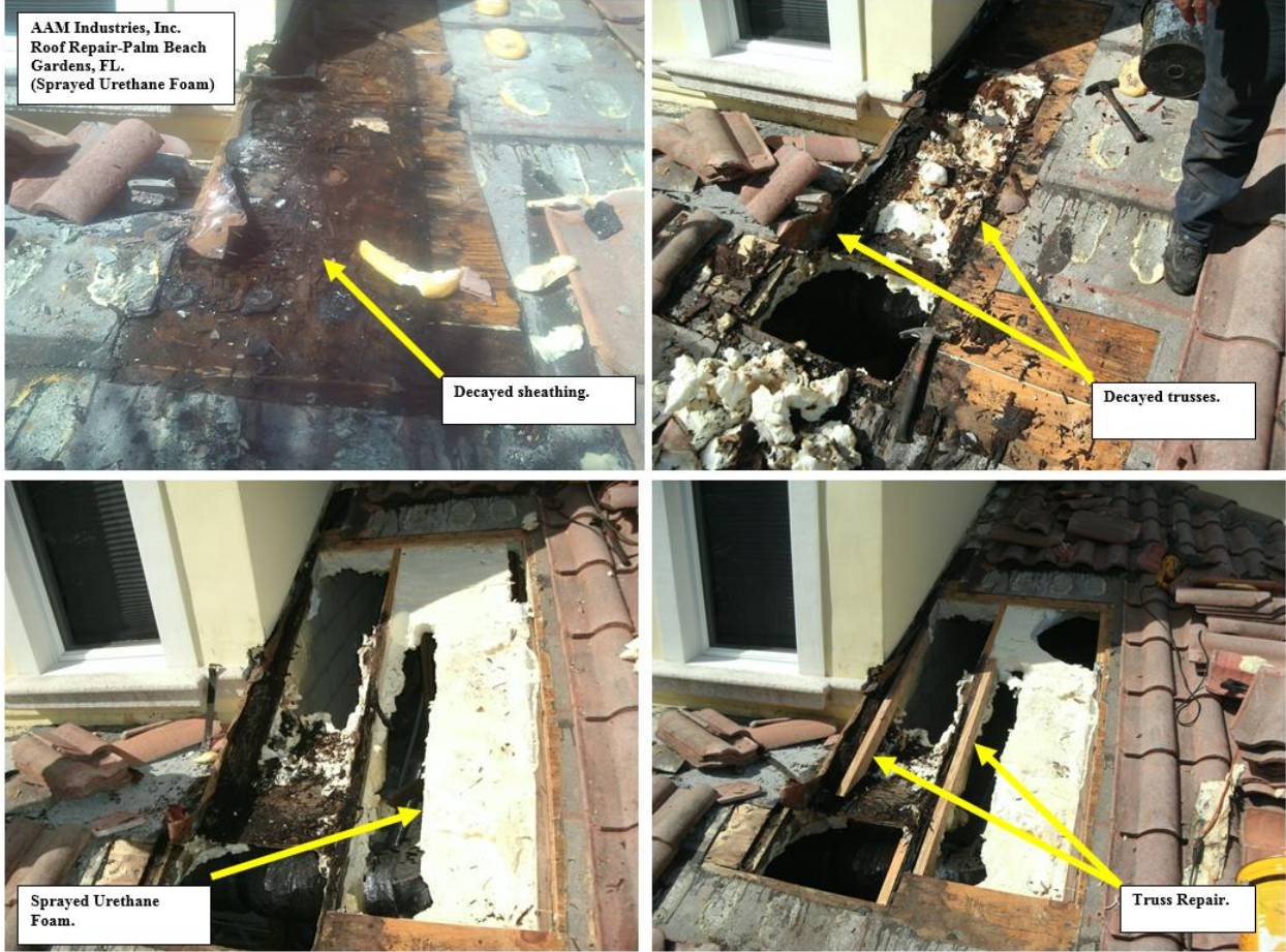
Figure 9: Moisture damage around a gable dormer to an unvented attic with ccSPF.
